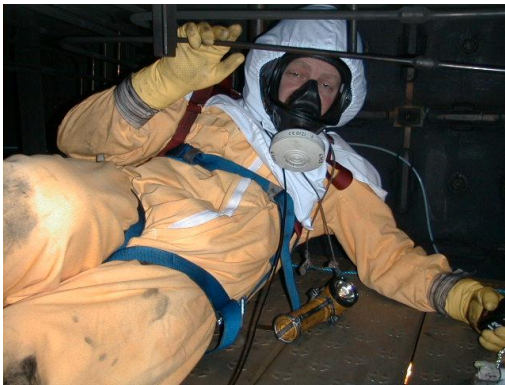
Protective clothing required for working within the Sub-Boiler Annulus
