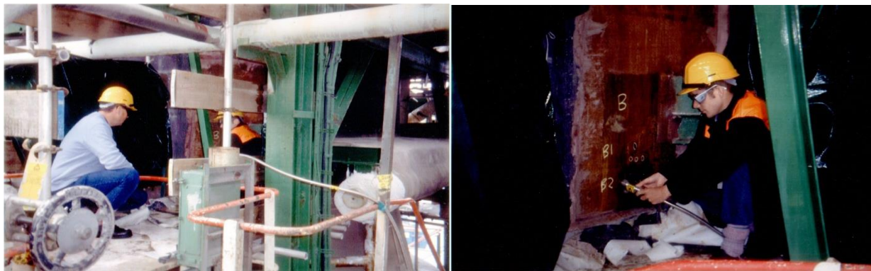
Deployment of the FO-LIBS instrument at Calder Hall nuclear power station
