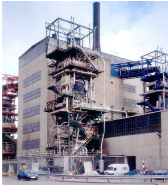
Calder Hall Magnox nuclear power station, Sellafield, UK
