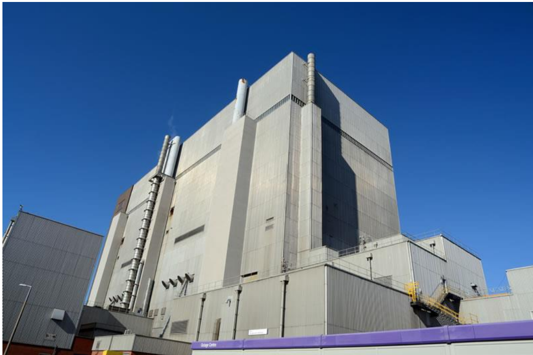
Heysham 1 nuclear power station, Lancashire, England
