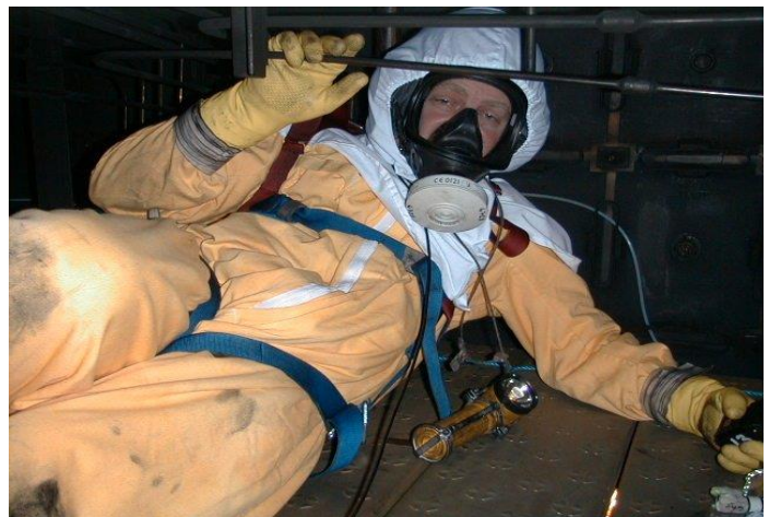
Economiser tubes located in the SBA (left). Protective clothing and equipment required for man-access to SBA (right)
