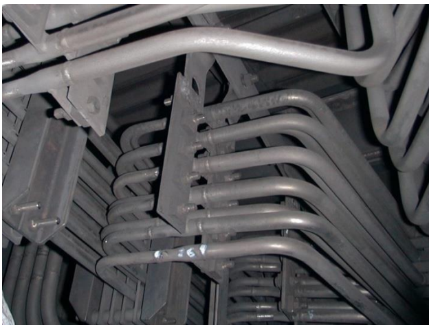
Economiser tubes located in the SBA (left). Protective clothing and equipment required for man-access to SBA (right)
