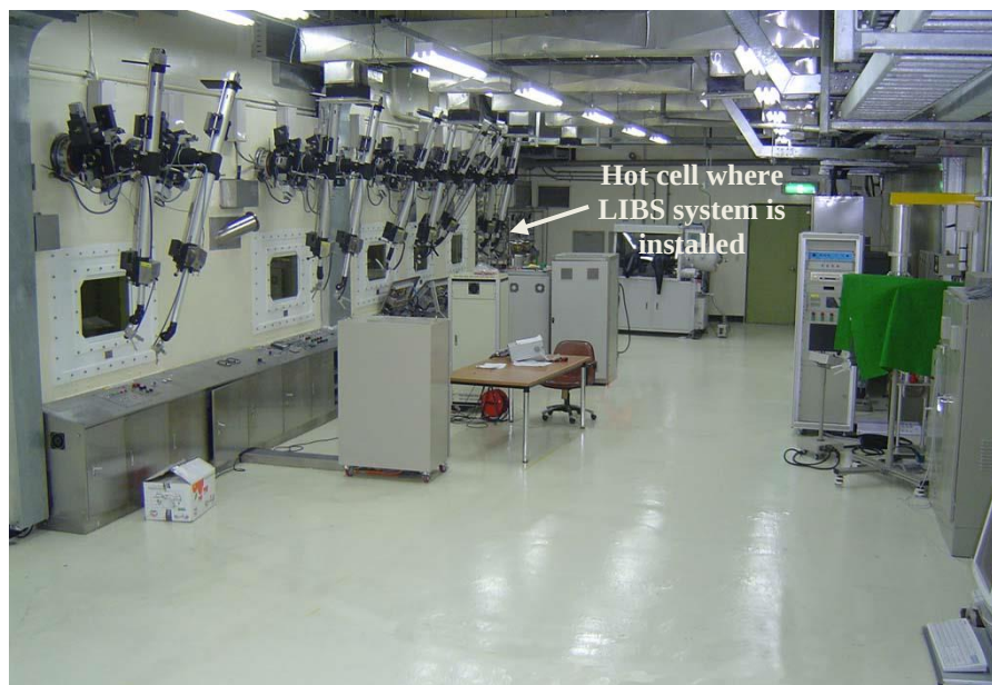
Image of IMEF hot cell facility highlighting the location of the LIBS system
