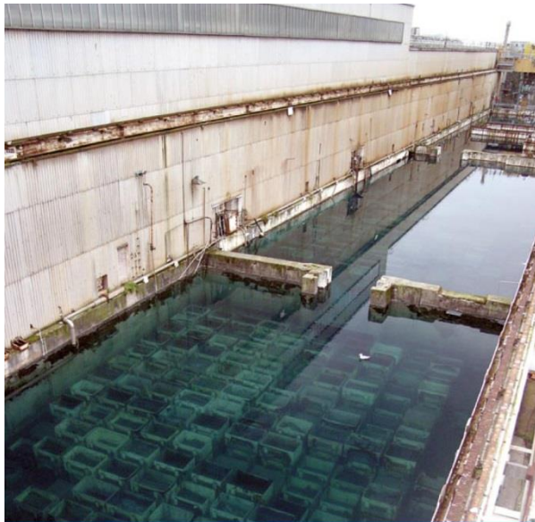
Typical early-design spent fuel cooling pond containing corroded fuel and waste materials
