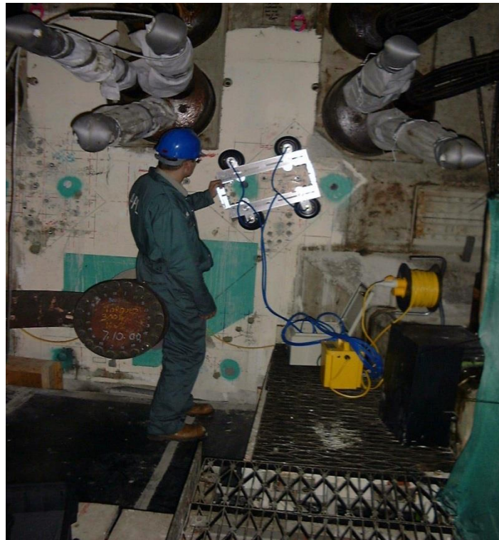
Testing of the heavy-duty vacuum cups used for attachment of the ST-LIBS module to the pressure vessel wall in the absence of suitable bolt anchor points
