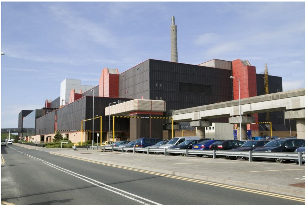
Thermal Oxide Reprocessing Plant (THORP), Sellafield, UK
